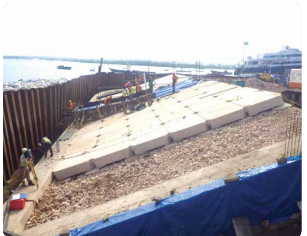
After starting construction works (March 2020)
