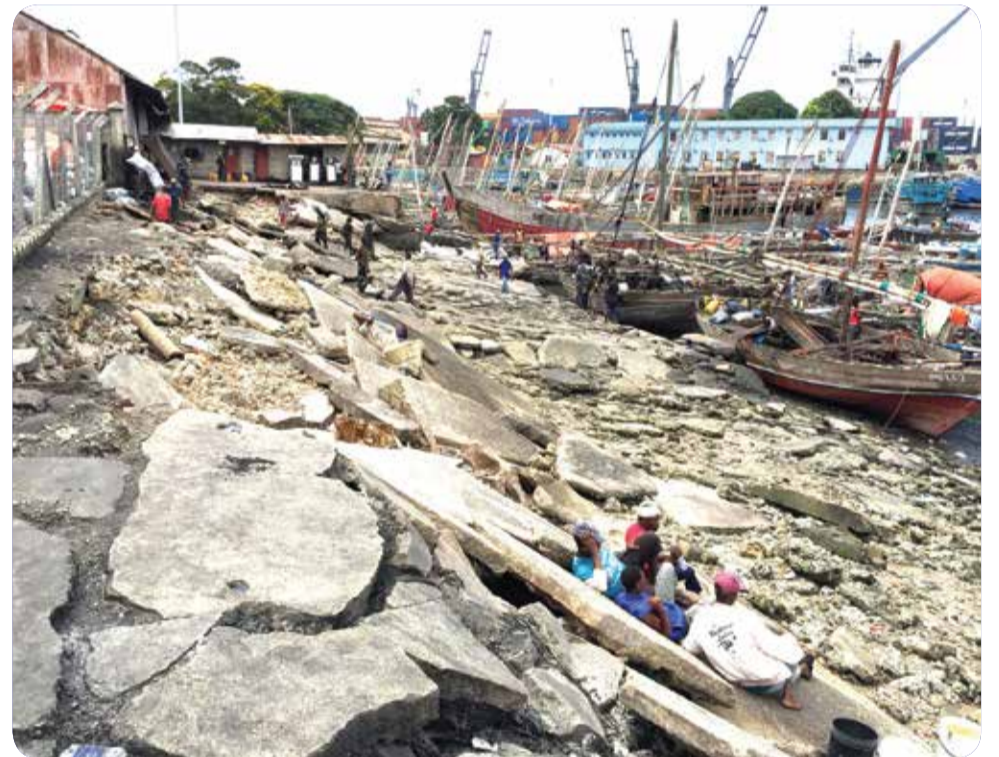
Before construction work (December 2015)
