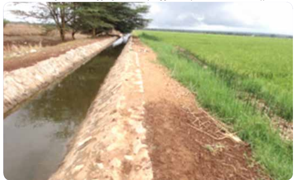
Completed repair work canal
