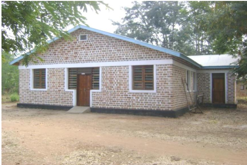
NEWLY CONSTRUCTED NSIMBO WARD OFFICE – MPANDA DC
