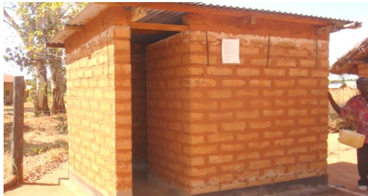
Sample Toilet with a Flier
