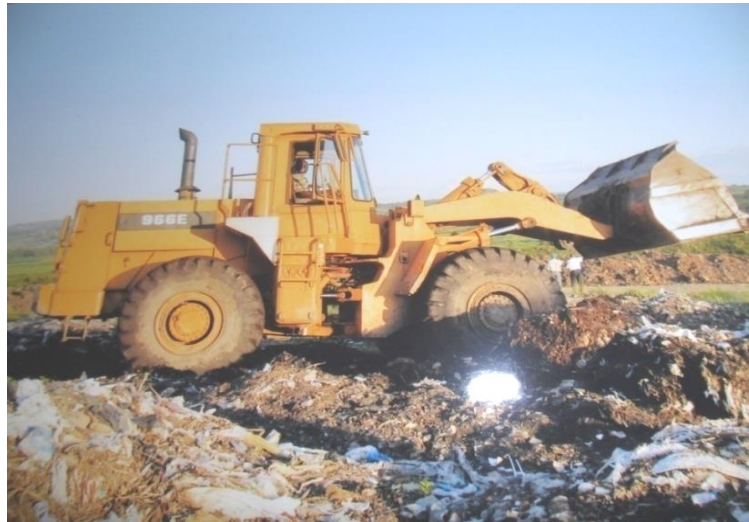
Hired wheel loader working at the landfill
