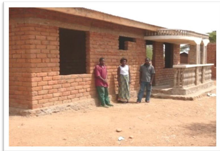
A Modern House under Construction
