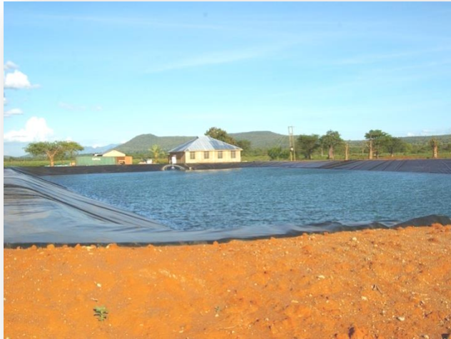
WATER DAM FOR IRRIGATION
