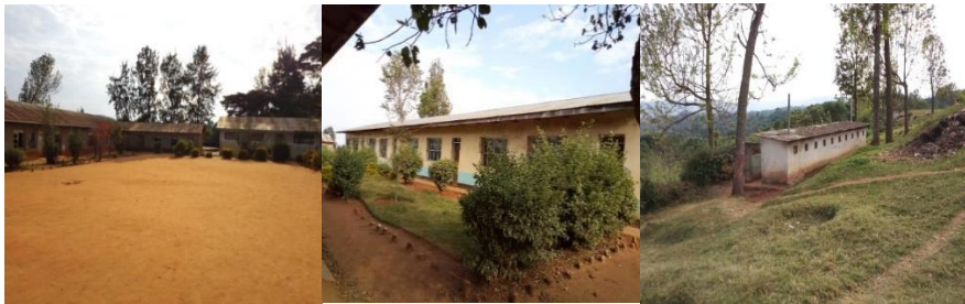
Murray Secondary School infrastructure
