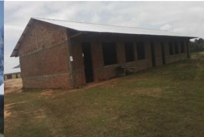
3 unfinished Science Laboratory rooms
