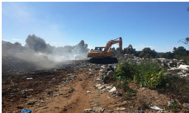
Excavator at Maheve dumping site
