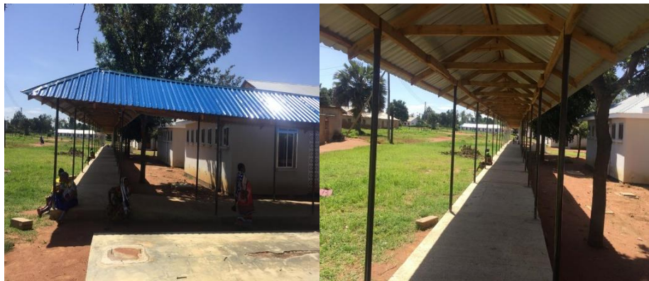
Walk ways constructed in Sokoine Health center
