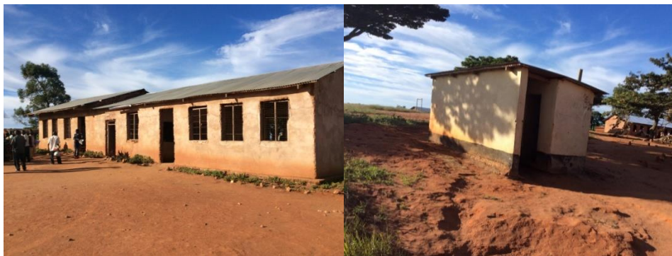
Matuli Primary School infrastructure
