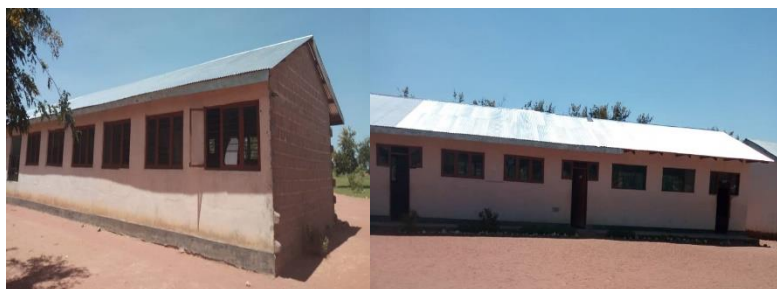
Renovated classrooms at Mtamaa Primary School
