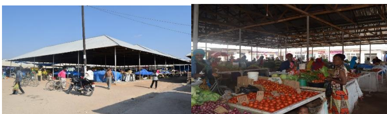
Front view of Main Market structure and stalls for vegetables vendors
