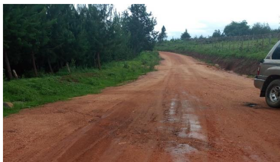
Upgraded Feeder Road to Matembwe Timber Market
