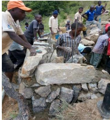
Construction work on progress
