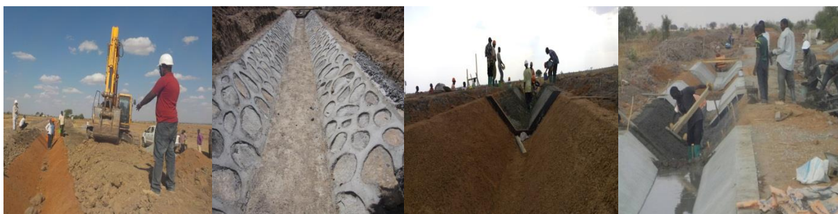
Canal construction works
