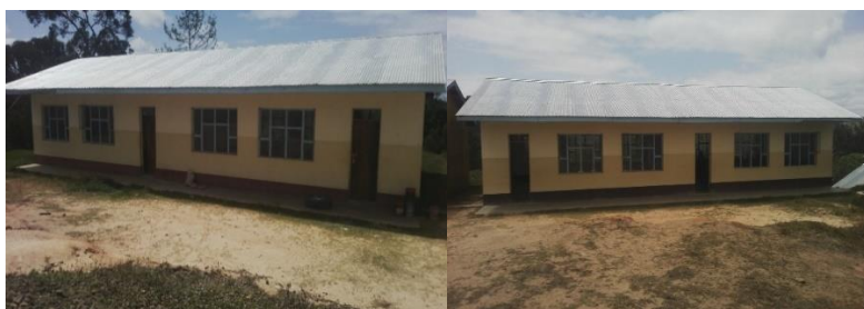
Four completed classrooms
