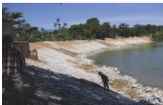
Low-cost small-scale river bank protection
