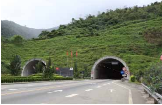
Hai Van Tunnel
