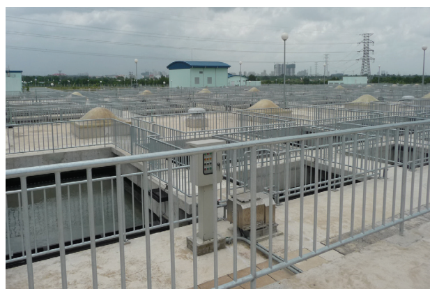
Ho Chi Minh City Water Environment Improvement (Wastewater Treatment Factory)
