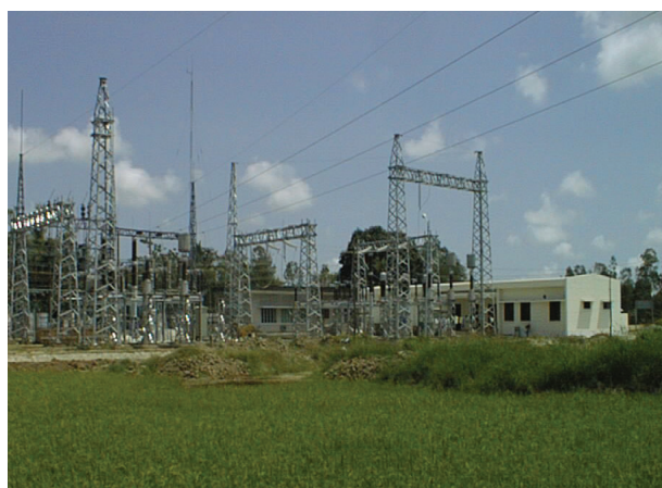
550KV Transmission line Phu My – HCM City constructed by yen loan
