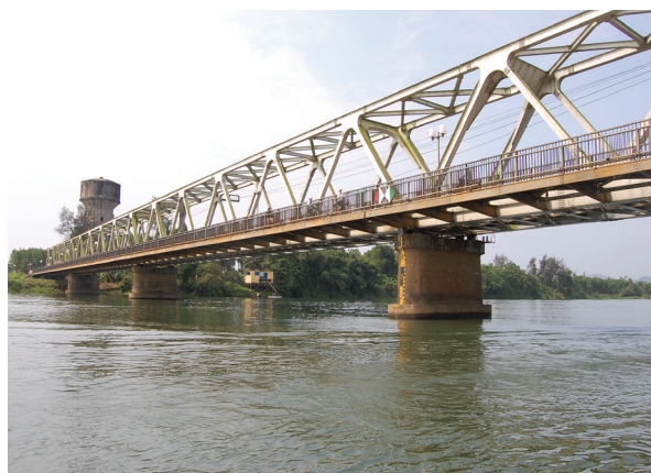
Bach Ho Bridge, Hue city (Rehabilitation of bridges along Hanoi – Ho Chi Minh City railway)
