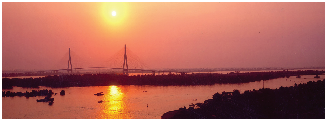
Can Tho Bridge
