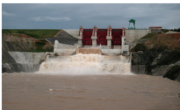
Dai Ninh Hydro Power Plant
