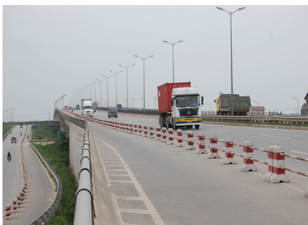
Thanh Tri Bridge
