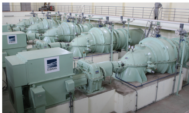
Yen So Pump Station
