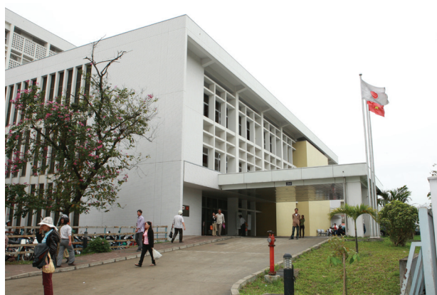
Improvement of Hue Central Hospital (Grant Aid)
