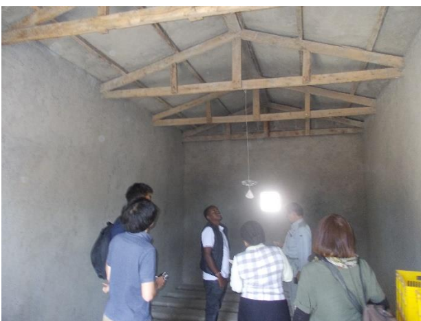
Potato-storage facility exterior (up) and interior (down).
