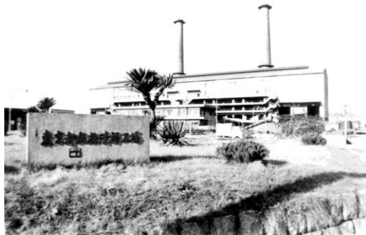
Photo 19 Itabashi Incineration Plant (Completed in 1961)
