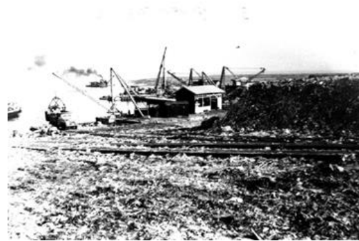
Photo 12 A Landfill Site in Tokyo where Spontaneous Combustion was Occurring Because the Waste was Directly Disposed with no Intermediate Treatment and no Soil Cover Application – circa 1957
