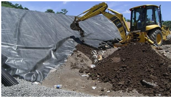
Photo 7-18 Practice of Applying Soil Cover
