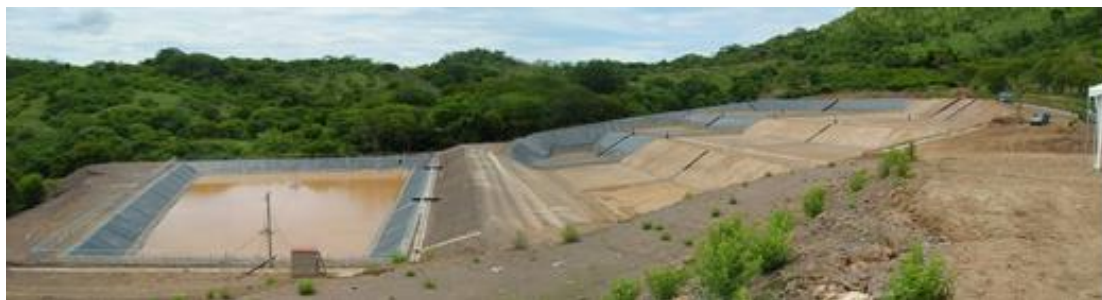
Photo 7-26 Newly Constructed Sanitary Landfill (Phase 2)
