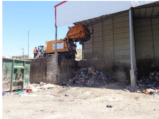
Photo 7-10 Hebron Transfer Station (Hebron JSC)
