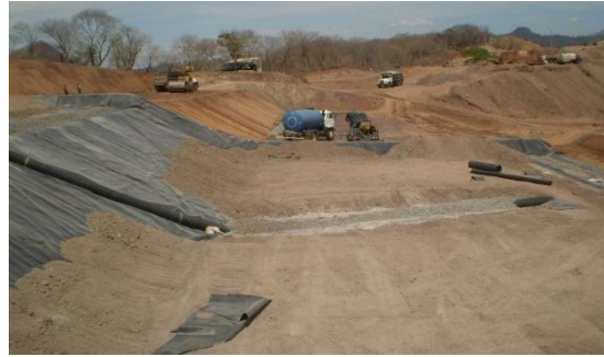
Photo 7-17 Sanitary Landfill under Construction (Phase2)
