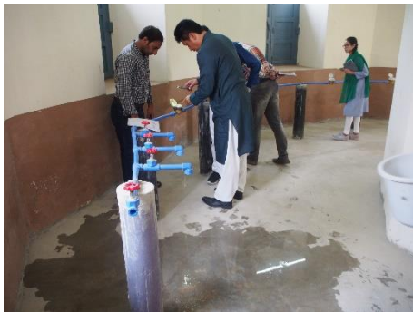
Construction of Simple Meter Workshop
