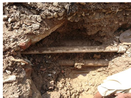
Situation of duplicated pipeline
