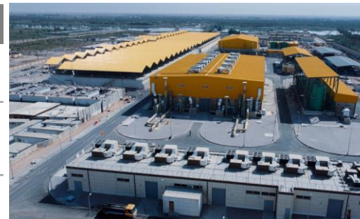
Newly constructed water treatment plants
