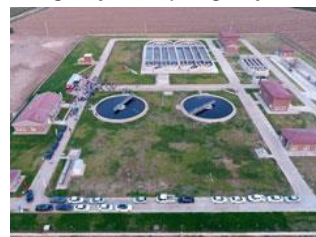
Sewage System (image by JICA)
