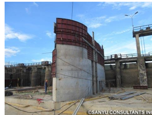
(Left photo) Tidal gate under construction (existing floodgate behind) (Upper right photo) The existing flood gate. Concrete and gate facilities are severely degraded (Bottom right of photo) Branch waterway that has been almost completely repaired
