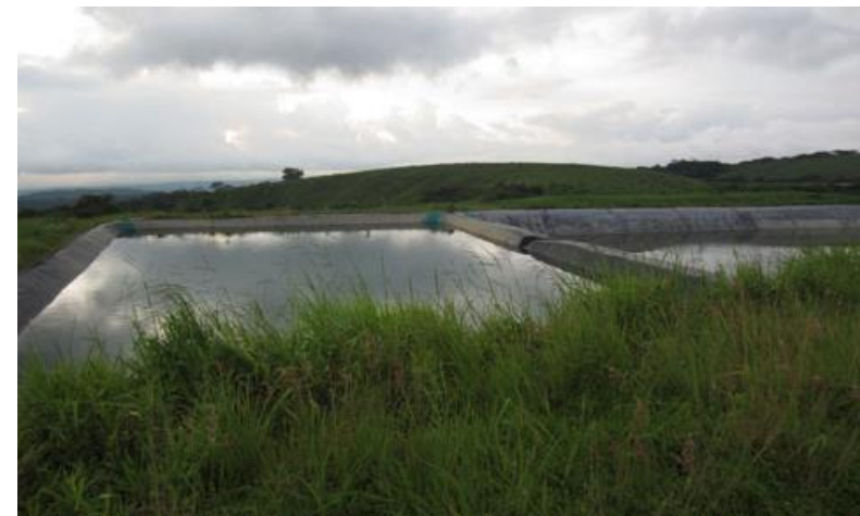
Guanacaste Geothermal Development (Before Use of Borinken 1 Hydrothermal Pit)
