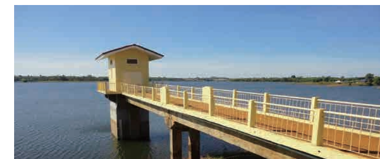
Water Intake Tower of O'Chum No.1 Dam
