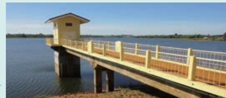
Water Intake Tower of O'Chum No.1 Dam
