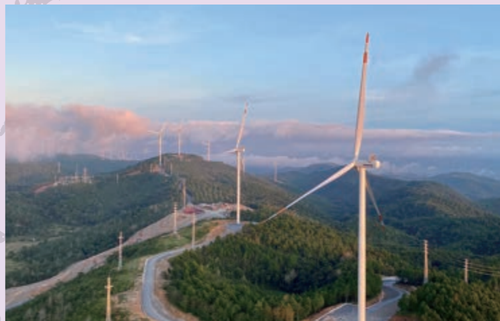
Turbines constructed under the project (Photo Credit : Power Construction Joint Stock Company No.1)
