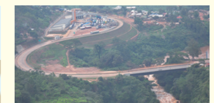
Rusumo International Bridge and One Stop Border Post Facilities (Tanzania and Rwanda)
