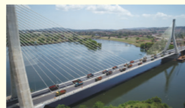
Source of the Nile Bridge (Uganda)
