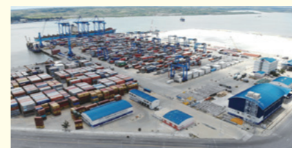
Mombasa Port Development Project and Mombasa Port Area Road Development Project (Kenya) [Photo: Toyo Construction Co., Ltd.]
