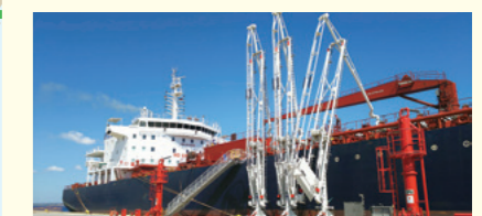
Nacala Port Development Project (Mozambique)
