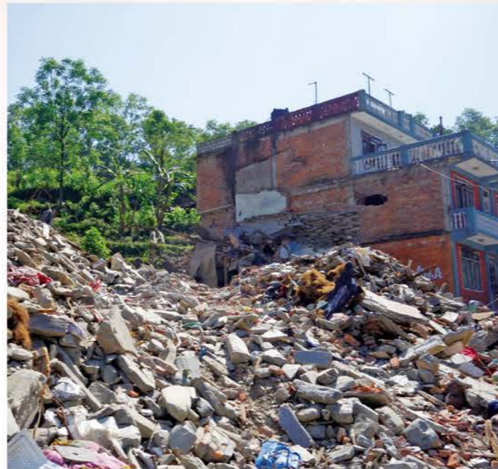
Examples of some buildings (in the back) that survived the earthquake by having, though inadequate, rebar and crossbeams. The collapsed private buildings did not have any reinforcements (foreground) (Nepal, May 2015)
