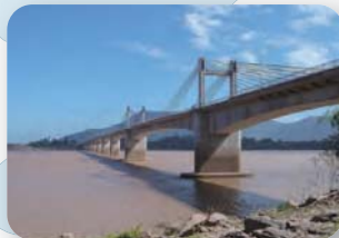
5 Pakse Bridge (Grant)
