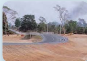
1 Bridge on Route 13 Rehabilitation (Grant)
