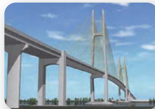
7 Neak Loeung Bridge (Grant)
