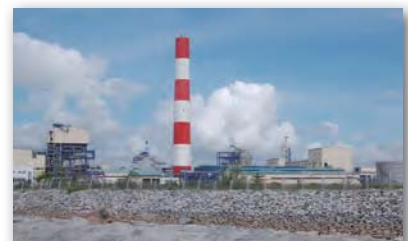
O Mon Thermal Power Plant in Vietnam
