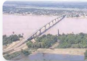
6 KIZUNA Bridge & National Road No.6-7 (Grant)
