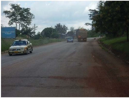
DBST on Western Corridor in Ghana
