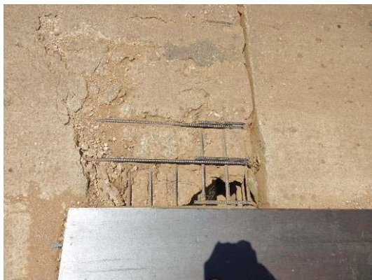
Buipe Bridge in Ghana
