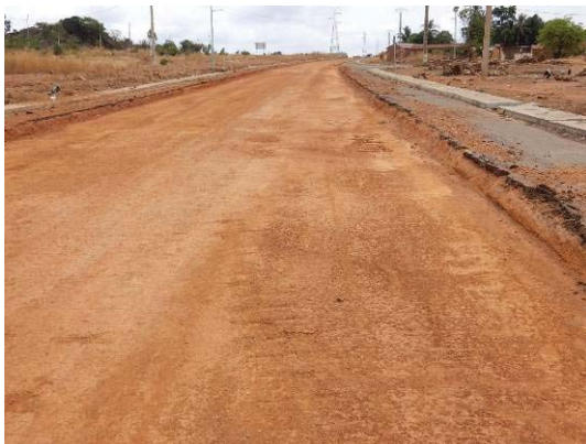
Bafilo Bypass in Togo
