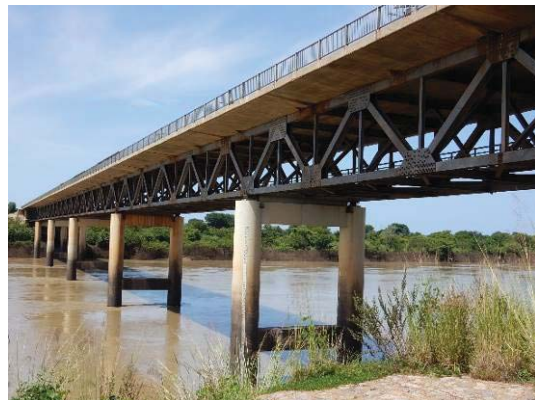
Yapei Bridge in Ghana
