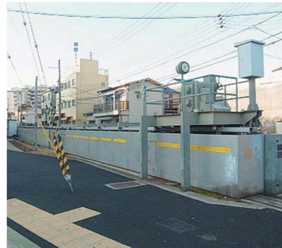
Seawalls in Kobe City's Chuo Ward
