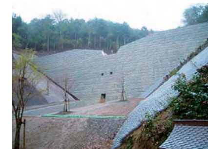
Soil erosion barrier for the prevention of landslides (Sasayama City)
