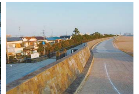
Seawall for the prevention of high tides (Nishinomiya City)
