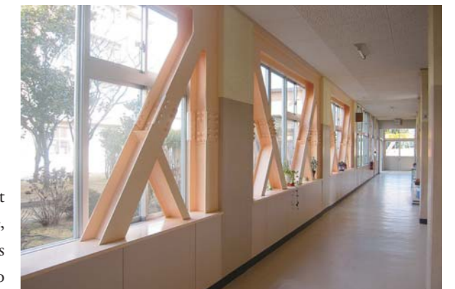
A seismically reinforced elementary school (Miki Municipal Hirono Elementary School)
