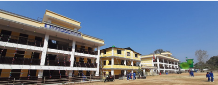
Complete view of the reconstructed buildings.
