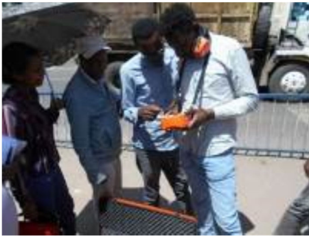
Photo 3 Confirmation of Correlative Leak Detector Handling Status
