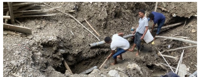
Photo 4 Pipe repair work
