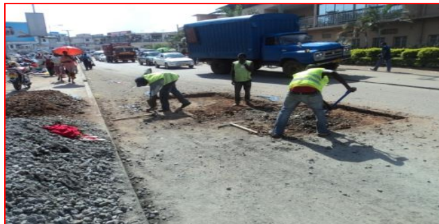
Road rehabilitation in progress
