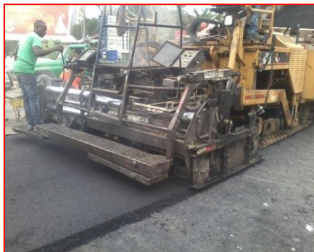
Construction of Pansiansi – Buzuruga road
