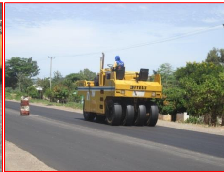
Asphalt rolling along Pansiansi – Buzuruga road
