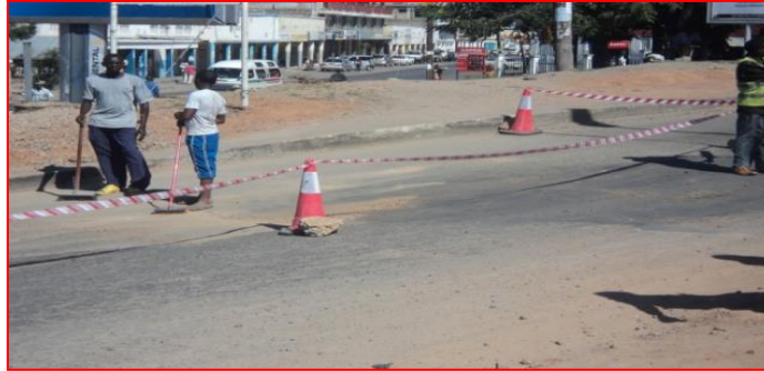
Cleaning of roads in progress
