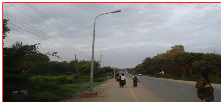
Street lighting along Mkuyuni Butimba road 2013/2014
