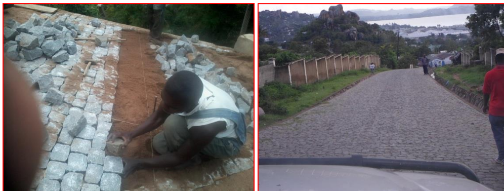
Stone paving of roads
