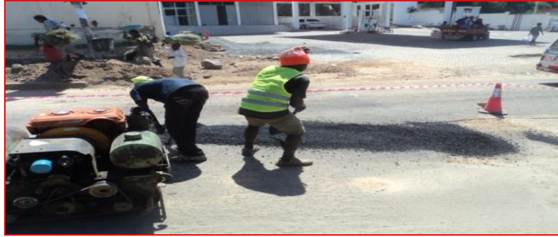
Patchworks along Pamba road on progress in 2012 using Council own funds
