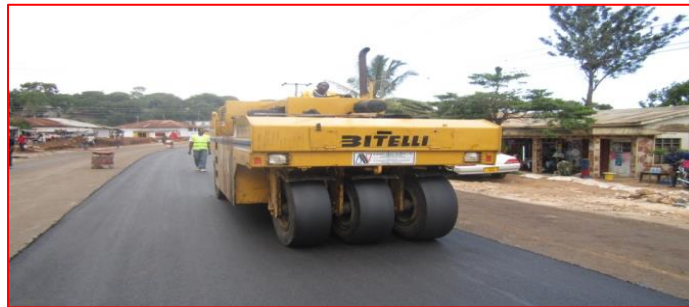
Construction of Pasiansi – Buzuruga 7.32km road in 2012 to Asphalt concrete standard
