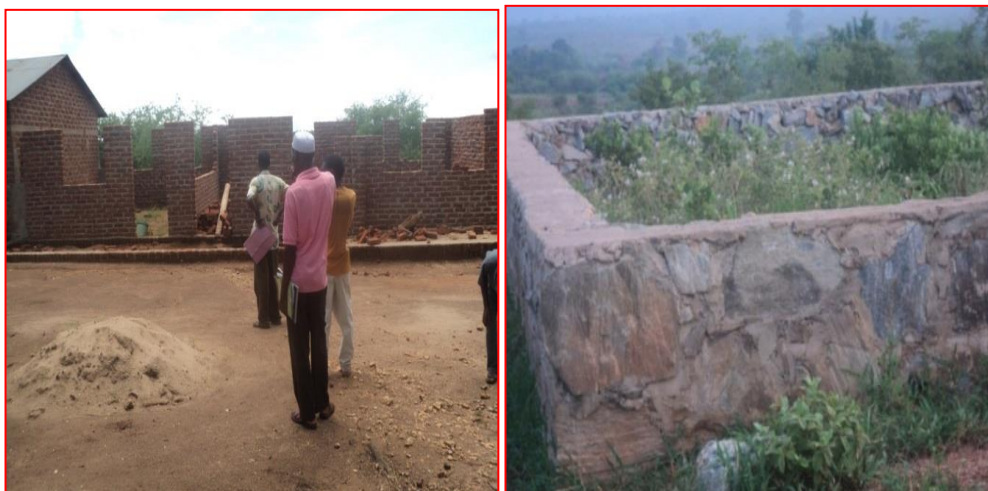
Construction of dispensary in Kinonko Village
