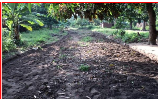
Feeder Road in Mangula-B village constructed using labor-based technology
