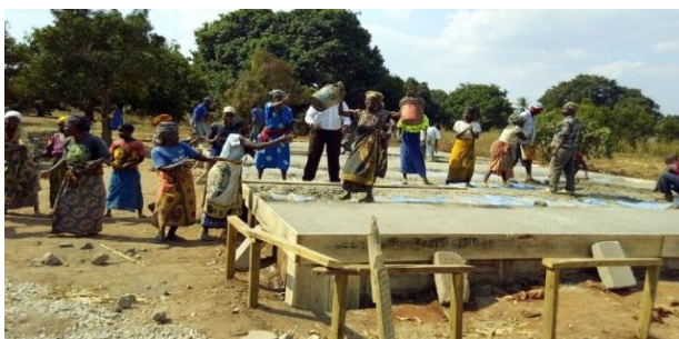
Community members participating in construction of classrooms
