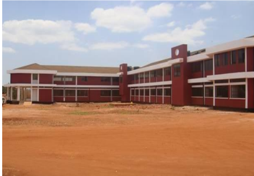
Nachingwea District Boma completed through stakeholders contributions
