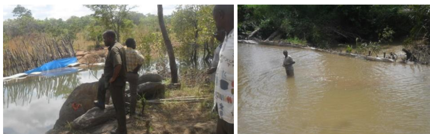
Traditional/local weir before Improvement at Kitanda and Legezamwendo Irrigation schemes
