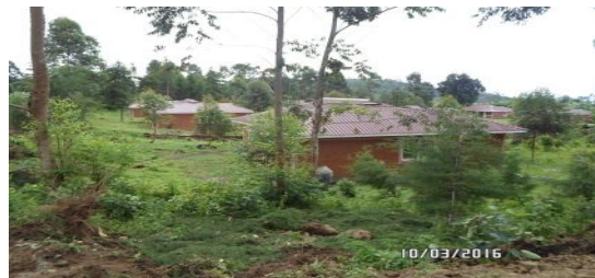
Acquired land for construction of Council staff houses
