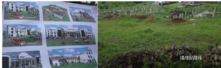
Proposed Council HQ and ongoing construction at foundation level
