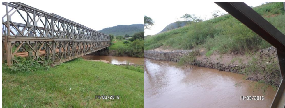
Rehabilitated Songwe River Bridge and banks
