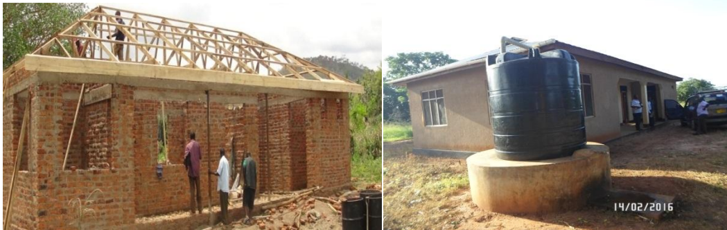
Construction of Kinyope village office and completed Likwaya Village office
