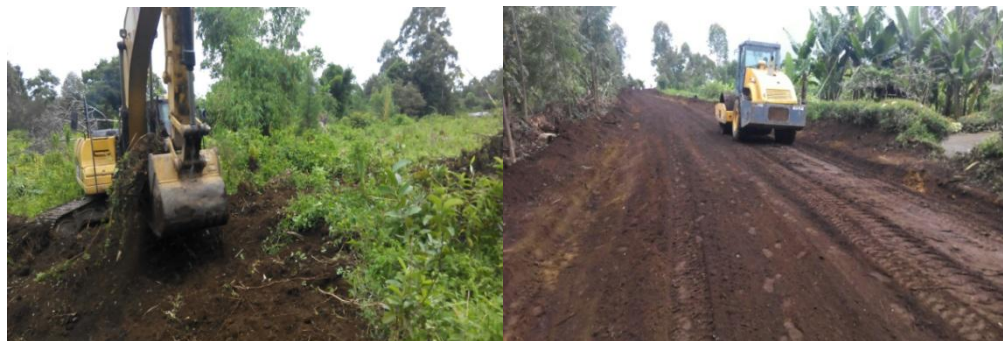
Excavated Mpanda to Market center access road
