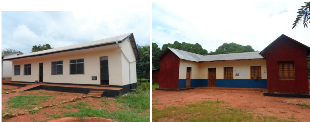
Classrooms at Nachingwea Girls’ S/School
