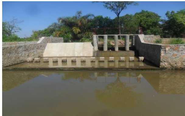
Constructed diversion intake at Kitanda Irrigation scheme
