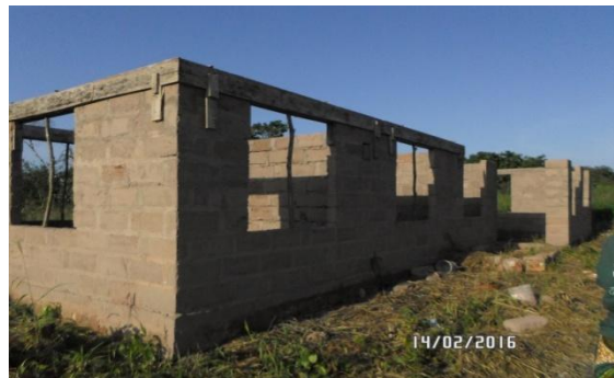
Teacher's house at Likwaya P/school under construction
