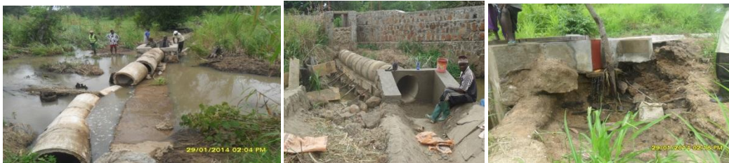
Rehabilitation of irrigation structures
