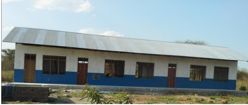
Three primary school classrooms, store and teachers' office built from the forest fees
