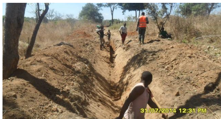
Ongoing excavation of irrigation canal in Madaba irrigation scheme
