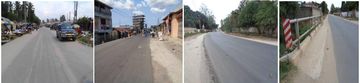
Tegeta market road 1km Tandale market road Journalism Road (1.1 Km) Feza Box Culvert – Mikocheni
