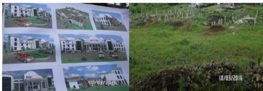
Proposed Council HQ and ongoing construction at foundation level
