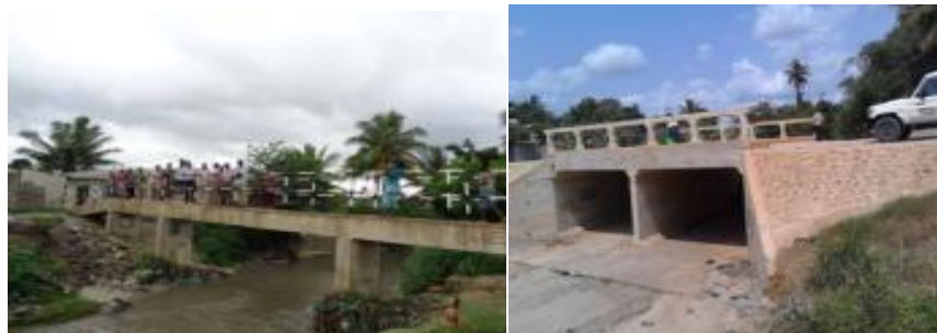
Pedalstals Bridge at Mburahati Ward and Msigani Bridge - Msigani Ward
