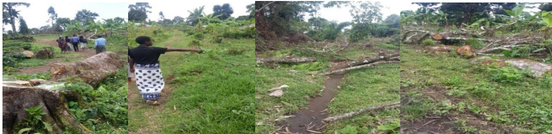
Existing footpaths before clearing and excavation
