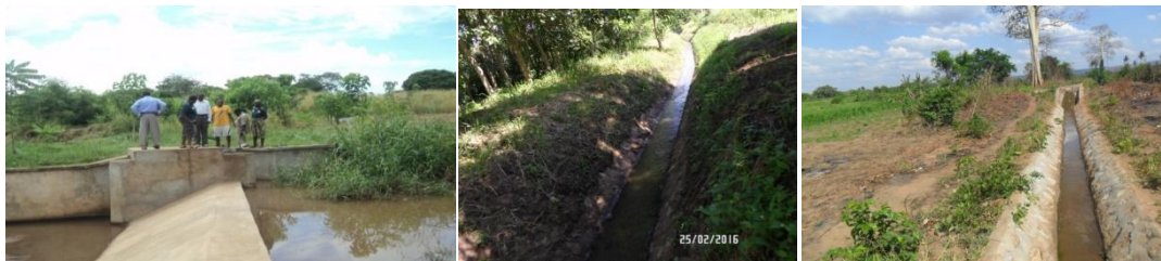
A well-constructed distribution box and two main canals
