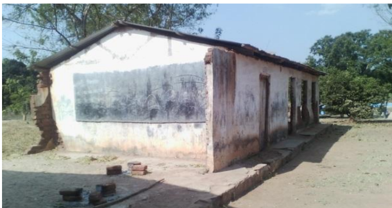
Old classrooms constructed by villagers for COBET Program
