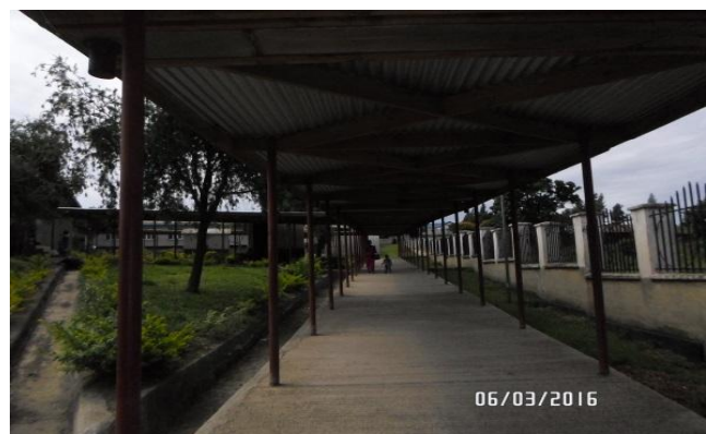
Storm water drainage and gardens
