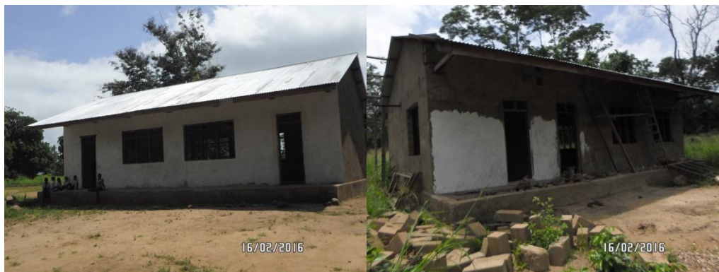
Two classrooms and a pre-primary class under construction at Nahanga Village
