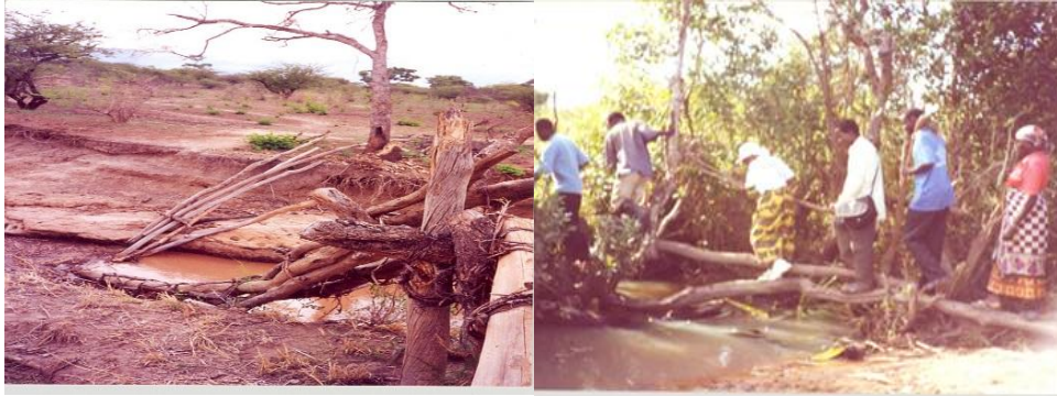
Blocked traditional bridge
