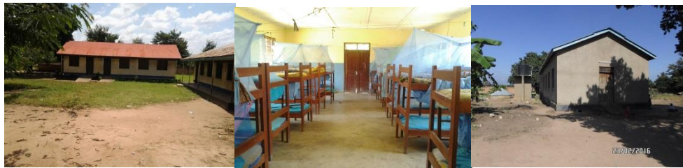
Classrooms and dormitory
