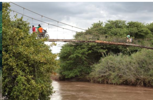
Kamsamba suspension bridge
