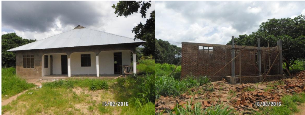
Constructed Dispensary and health staff house under construction
