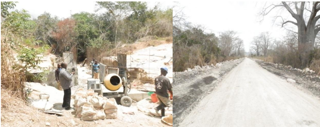
Construction works, Mvuleni – Kitomanga road during construction
