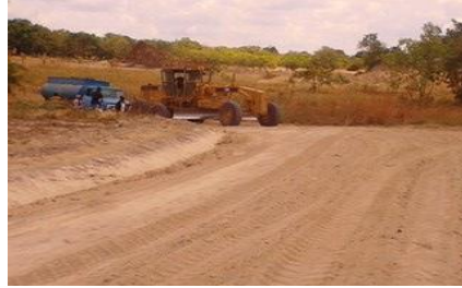
Feeder road constructed
