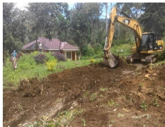
Council's Houses to Lwangwa Access Road
