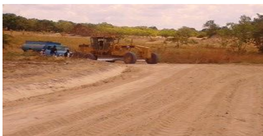
Ongoing construction of Lekindo Madaba road
