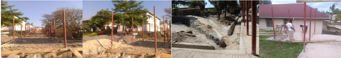
Ongoing construction of walkways
