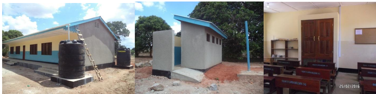
Two classrooms and a toilet (with 4 stances) constructed under TASAF support
