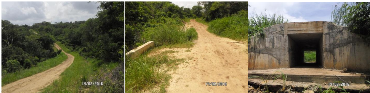
Mvuleni-Kitomanga road and bridge
