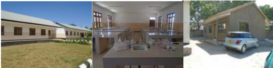
Laboratories and teacher' house constructed
