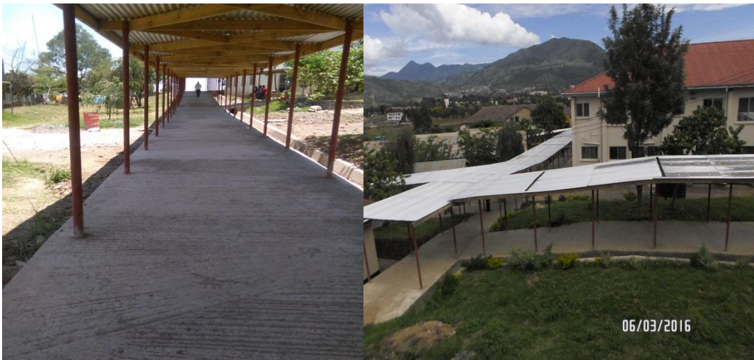
CONSTRUCTION OF HOSPITAL WALK WAYS
