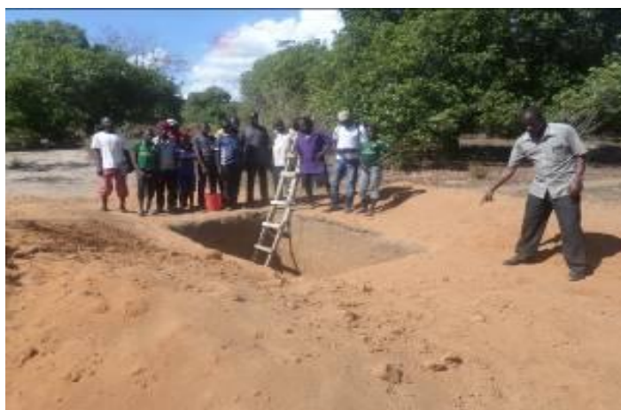
Mapili villagers participating in construction works
