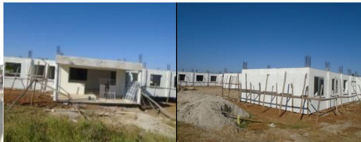
Mabwepande OPD and maternity hospital
