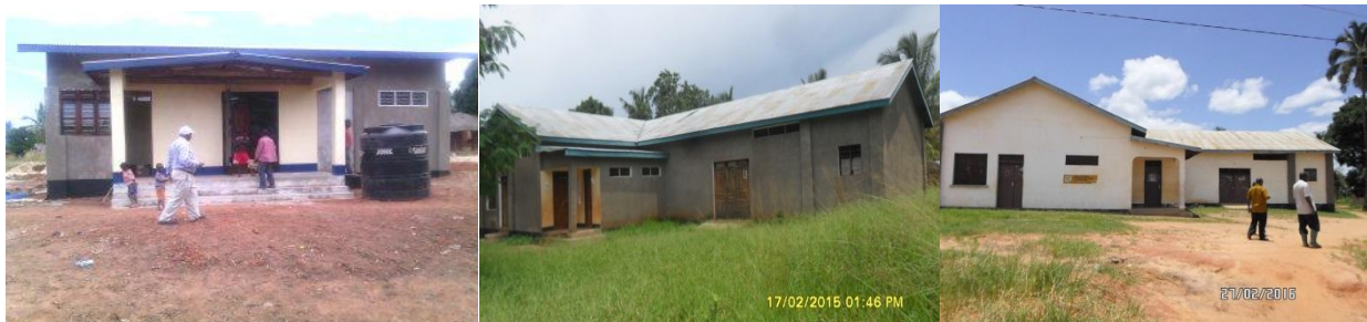
A warehouse built at Chingulungulu Village.
