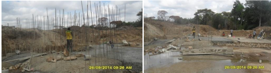
The ongoing construction of intake at Legezamwendo and Madaba irrigation schemes
