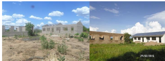
Construction of Chikoropola Ward Secondary school
