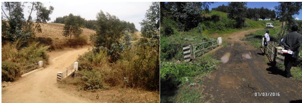
The Nkunywa Bridge during dry and rainy season
