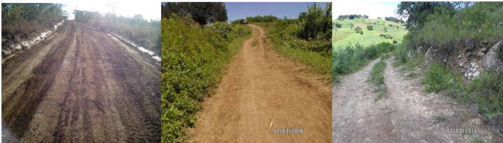
Road sections along Ntangano – Ijombe – Itewe Road
