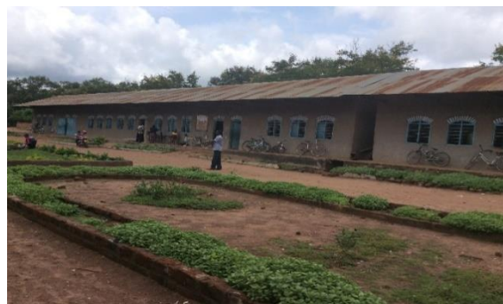
Msakila Primary School Infrastructure
