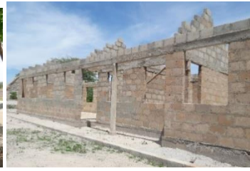
Laboratories under construction
