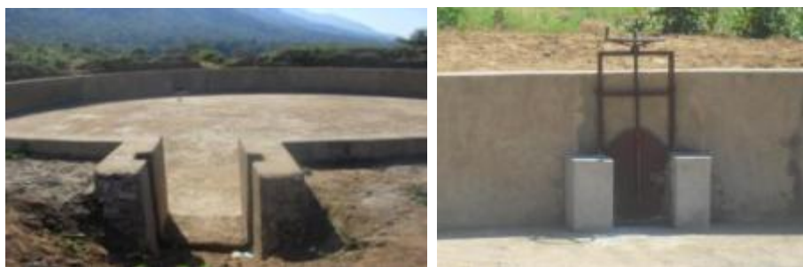
Water resevour and outlets at Sakalilo Irrigation Scheme
