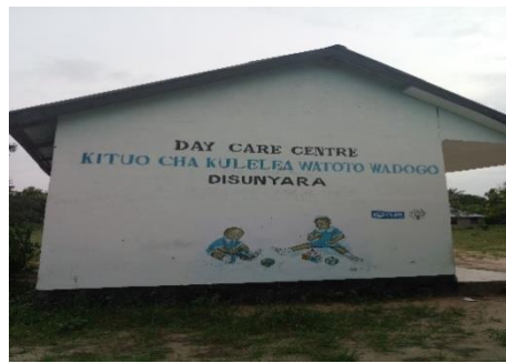
Disunyara day care center
