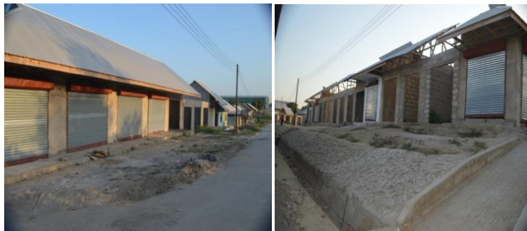
The newly constructed shops at Mnarani Market
