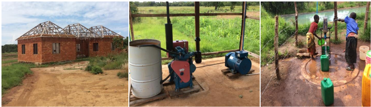
Office building, Workshop and water well
