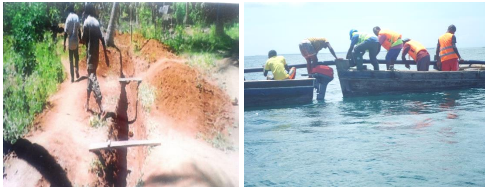
Digging of trenches and installation of water pipes across the ocean
