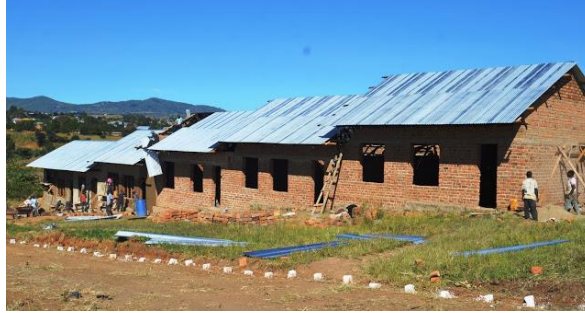
Extension of Kasiwe Primary School
