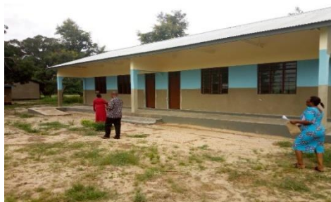
Newly constructed classrooms
