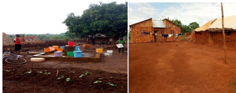
New brick-house under construction (left) and completed brick- house (right)
