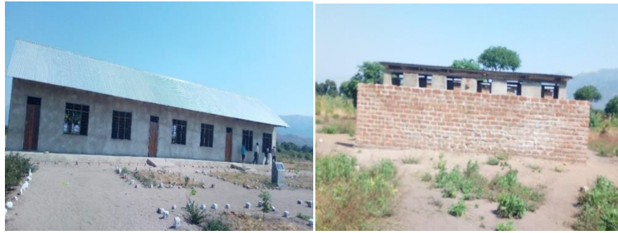
New classrooms and toilets of Mkuyuni Primary School
