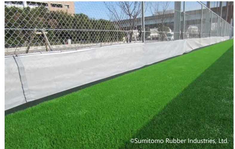
Installation of Mesh Net around the Field to Prevent Leakages of Artificial Turf
