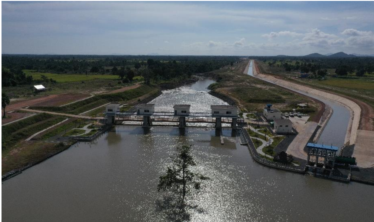
Headwork and Main Canal at Lum Hach Subproject of Kampong Chhnang Province
