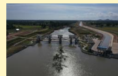
Headwork and Main Canal at Lum Hach sub-project of Kampong Chhnang province
