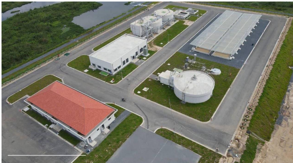
Cheung Aek Sewage Treatment Plant
