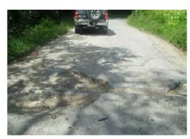
A road damaged by installation of water pipes
