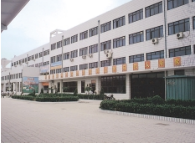
Hengshui Railway Station Building
