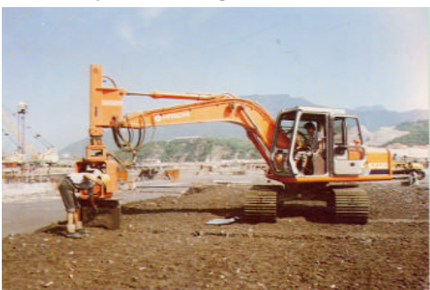
Step 3 Prepare lateral joints using a joint forming machine
