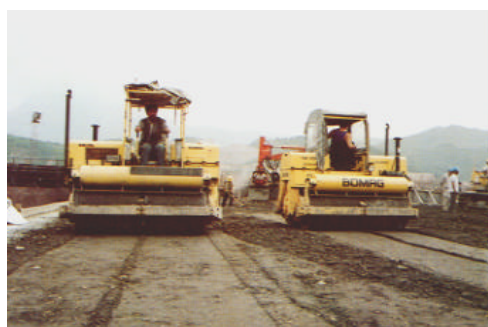
Step 4 Compact with rollers
