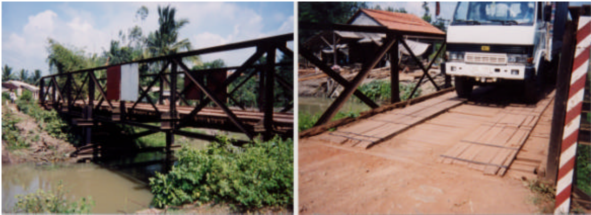
Photos 2 and 3 Dilapidated bridges on roads improved under this project (a side view of the bridge on the left and a truck crossing the same bridge on the right)
