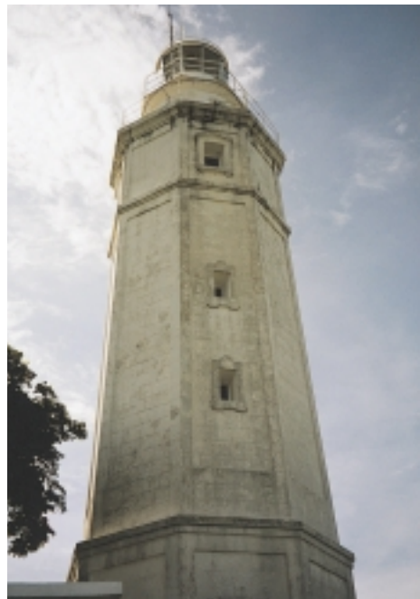
BAGACAY Light House
