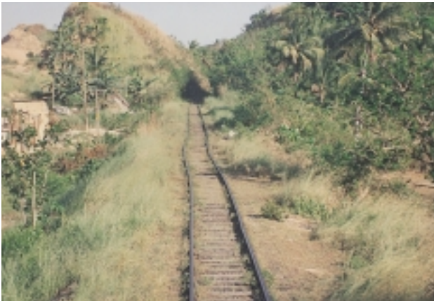
Railway Track(1993) before the Project : Implementation with Superannuated Ties and Bent Rails
