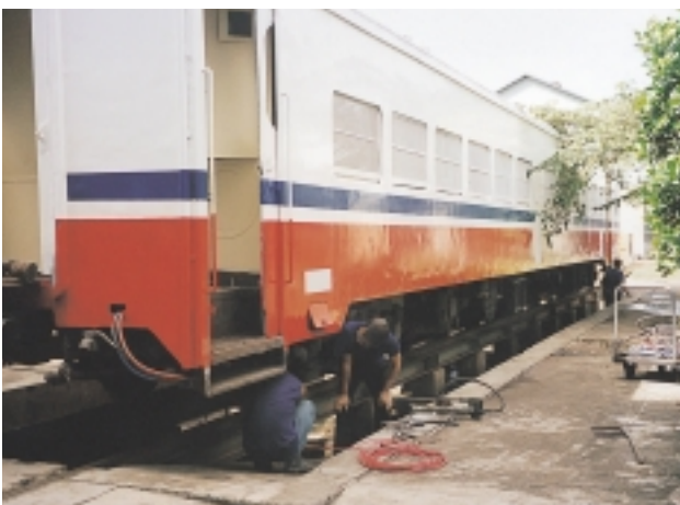
Rehabilitation Works on a Passenger Coach
