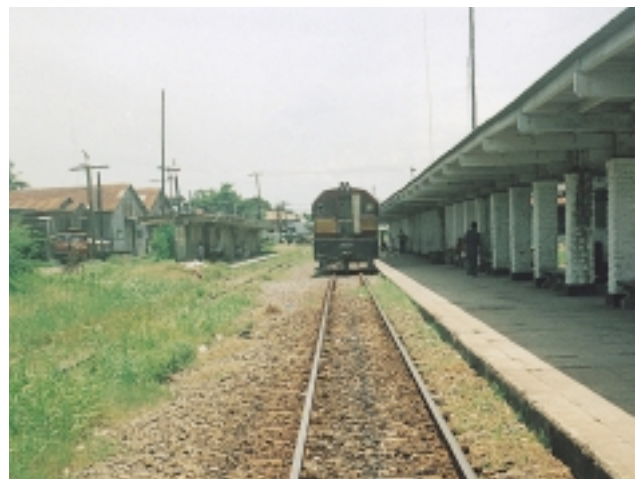
The Rehabilitated Track after this Project
