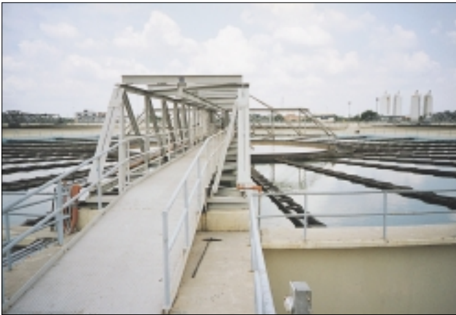
Bang Ken Water Treatment Plant expanded by this Project
