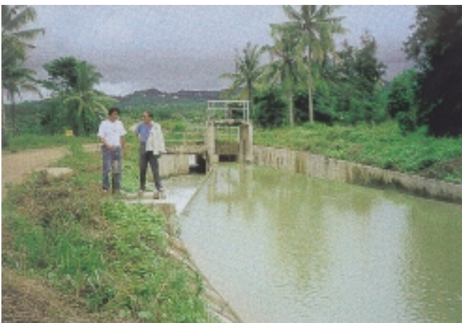
Sluice Gate in Main Canal
