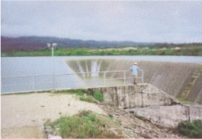
Malinao Dam Spillway
