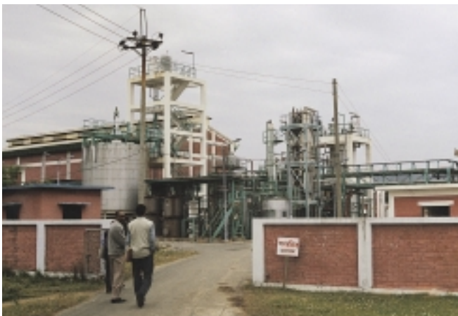
Plant Facilities after Renovation
