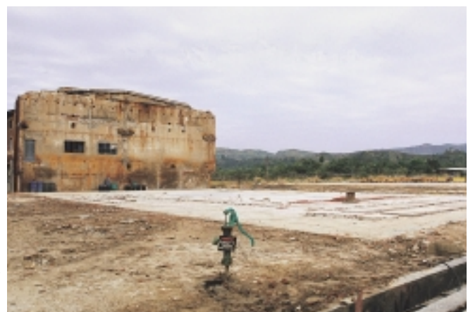
The Site of the Former Plant. Tube Well in the Picture is serving for Mercury Monitor The Processing and Recovery (decontamination) of Residual Mercury has been completed.
