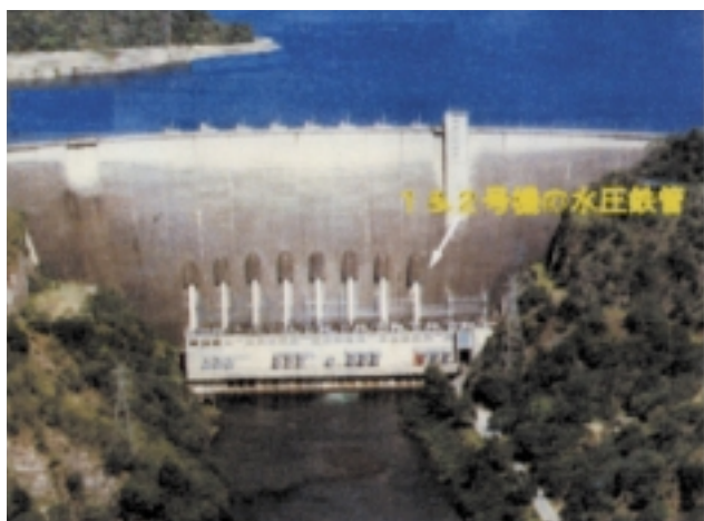
The Hydraulic Pressure Pipes, units 1 and 2
