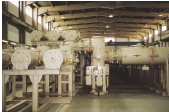
Gas Insulation Switchgear
