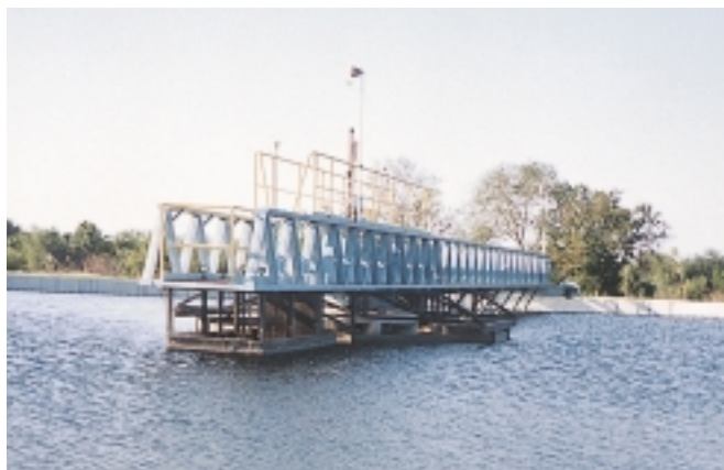
Secondary Sediment Facility of Noreste Water Treatment Plant
