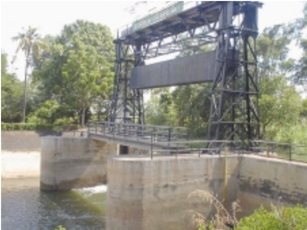
Sluice Gate on Lake Bung Borapet (Completed in 1992)
