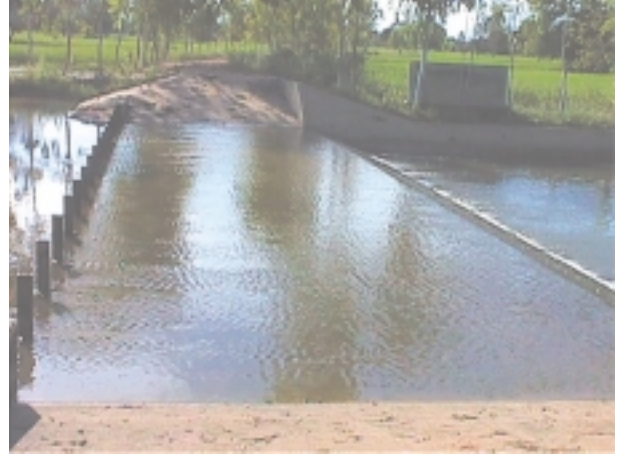
Ban Muang Noi Weir Facility
