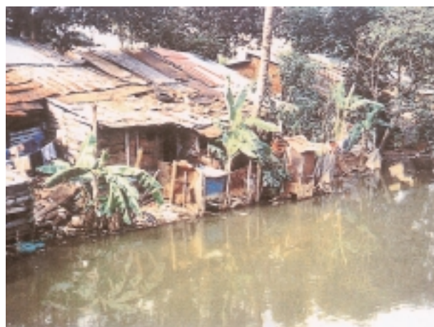
Shanty along the Dehiwala Canal (Before the project implementation)
