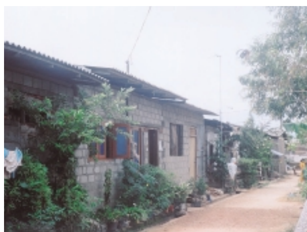
Badowita Area, One of the Resettlement Zones
