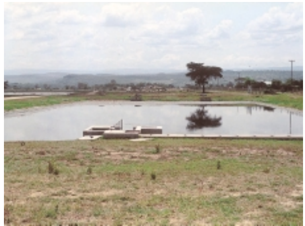
Njoro Sewage Treatment Works
