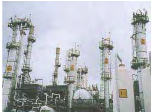
Introduction Facilities : HDD Equipment in Tula Oil Refinery
