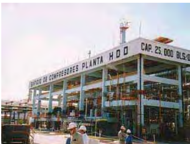
Introduction Facilities : HDD Equipment in Salamanca Oil Refinery
