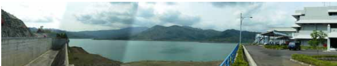
Figure 1. View of Wonorejo Multipurpose Dam
