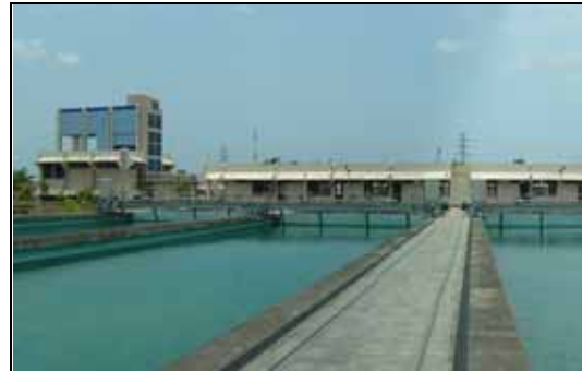
Water treatment facilities (settling tanks)
