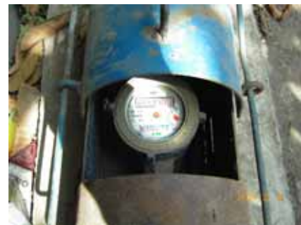
Fig. 3: One of the replacement water meters
