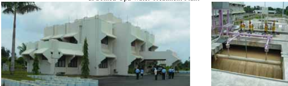
Fig. 4: Administrative buildings (left) and the raw water intake unit (right) at Somba-Opu Water Treatment Plant
