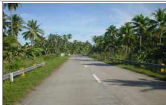
One of the arterial roads improved via the project
