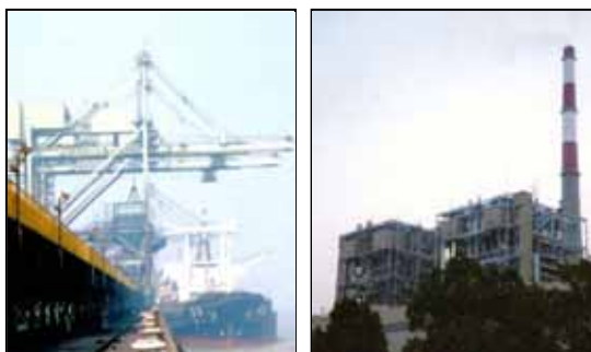
The berth (left) and power generator (right) constructed under the project
