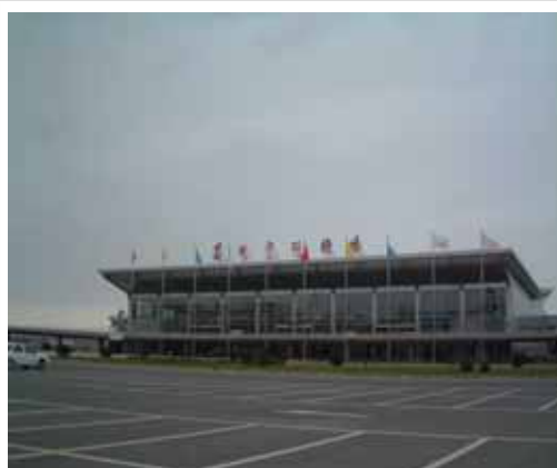
Lanzhou Zhongchuan Airport Terminal Building
