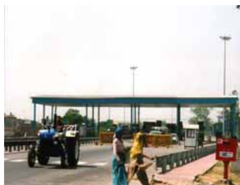
Figure 4: Toll booth on the project road
