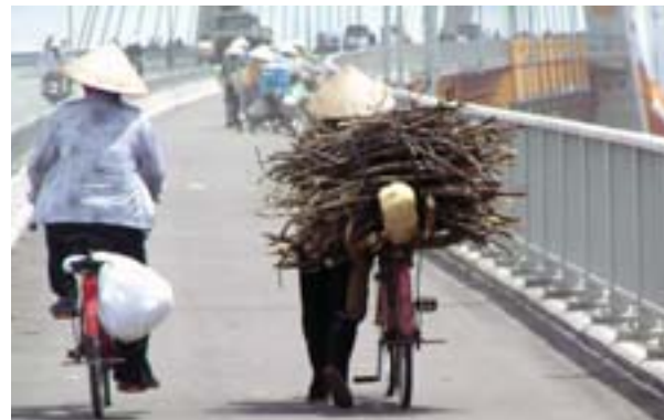
Vietnam’s Binh Bridge Construction Project for which a mid-term review was undertaken in FY2004
